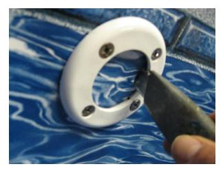
The return fitting face plate is installed in somewhat the manner as the skimmer. First find the round face plate and the pack of four faceplate screws supplied with the fitting. Note: there is <u>no</u> gasket installed between the liner and the return face plate. Press your
