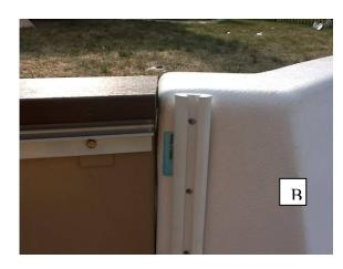
First locate the stair placement at the site. Align the appropriate panels to either side of the stair and clamp them to the stair flange. When using the "synthetic wood" top seat or the "PVC coping", the coping must be flush with the top of the stair as shown in photo B. see pages 12-15 for coping instructions
