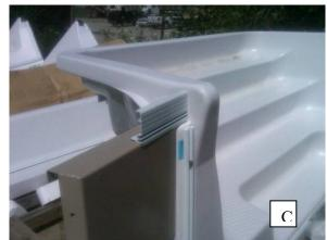
finished elevation is established, drill through the stair flange at each panel hole location using a 5/16" drill bit and bolt the panel to the stair.
