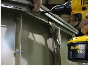
section of "J" channel is held on by four (4) of the self drilling self tapping hex read screws. Note: The slotted holes in the "J" channel are not used for this application.
