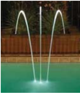
Laminars are more dramatic when the laminars are placed with the water flow aimed towards the main viewing area.
